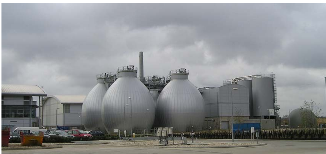
Egg shaped anaerobic digesters at Thames Water's Reading WwTW © Dr. Tim Evans, Tim Evans Environment
