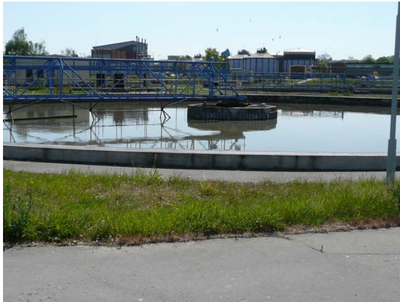
Primary settlement at Prague WWTW © Dr. Tim Evans., Tim Evans Environment
