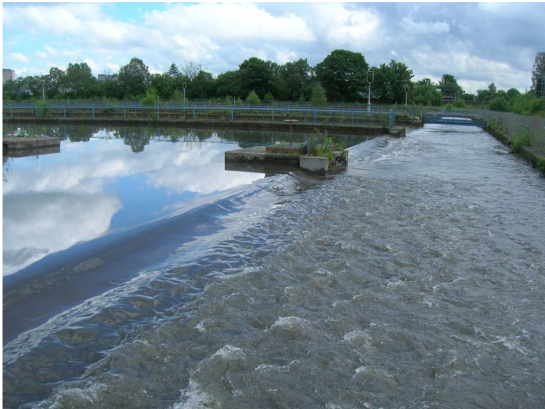
Figure 7: Storm tanks and outlet channel
