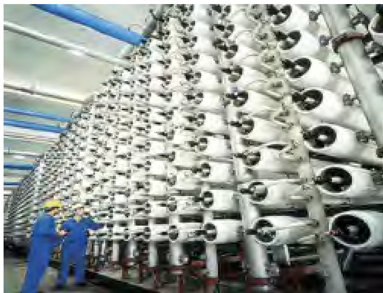
Figure 22: RO modules in a large desalination plant.
